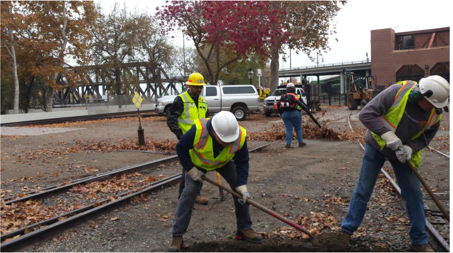
Work begins at Switch 3, the Stub-switch. The two Steves are digging out the crib and trench while Heather hurricanes away dead leaves
