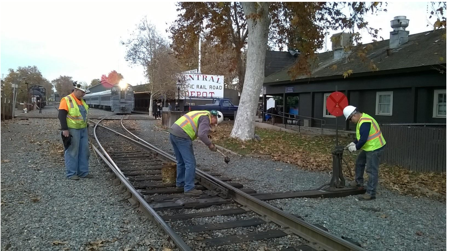
Servicing switches: Steve N. greases the switch-plates while Steve W. prepares to rotate the switch to "rub-in" in the grease
