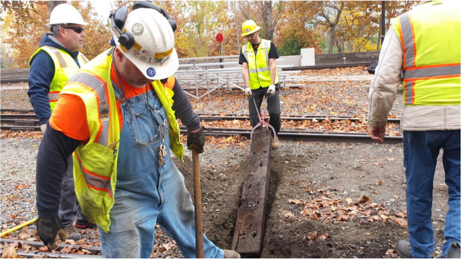
Mike F. and Chris pull the old rotten tie out
