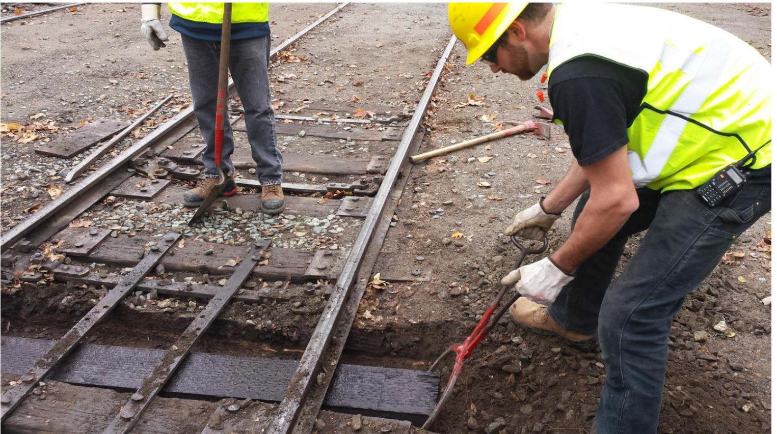
Chris pulls the new tie into place
