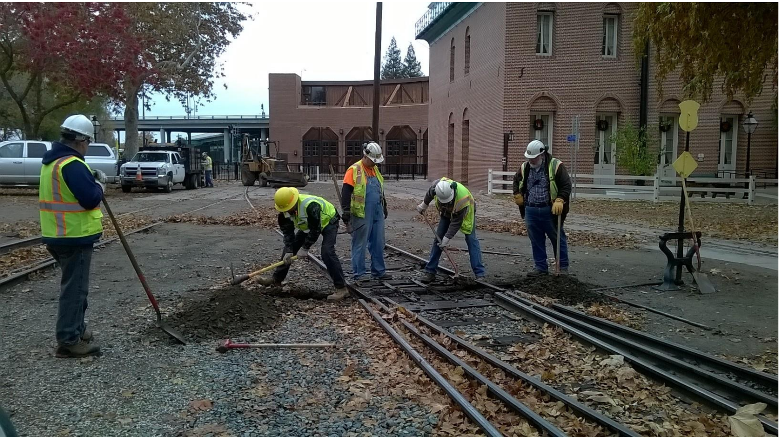
Steve W., Chris, Mike F., Steve N., and Frank continue digging out the tie cribs at Switch 3
