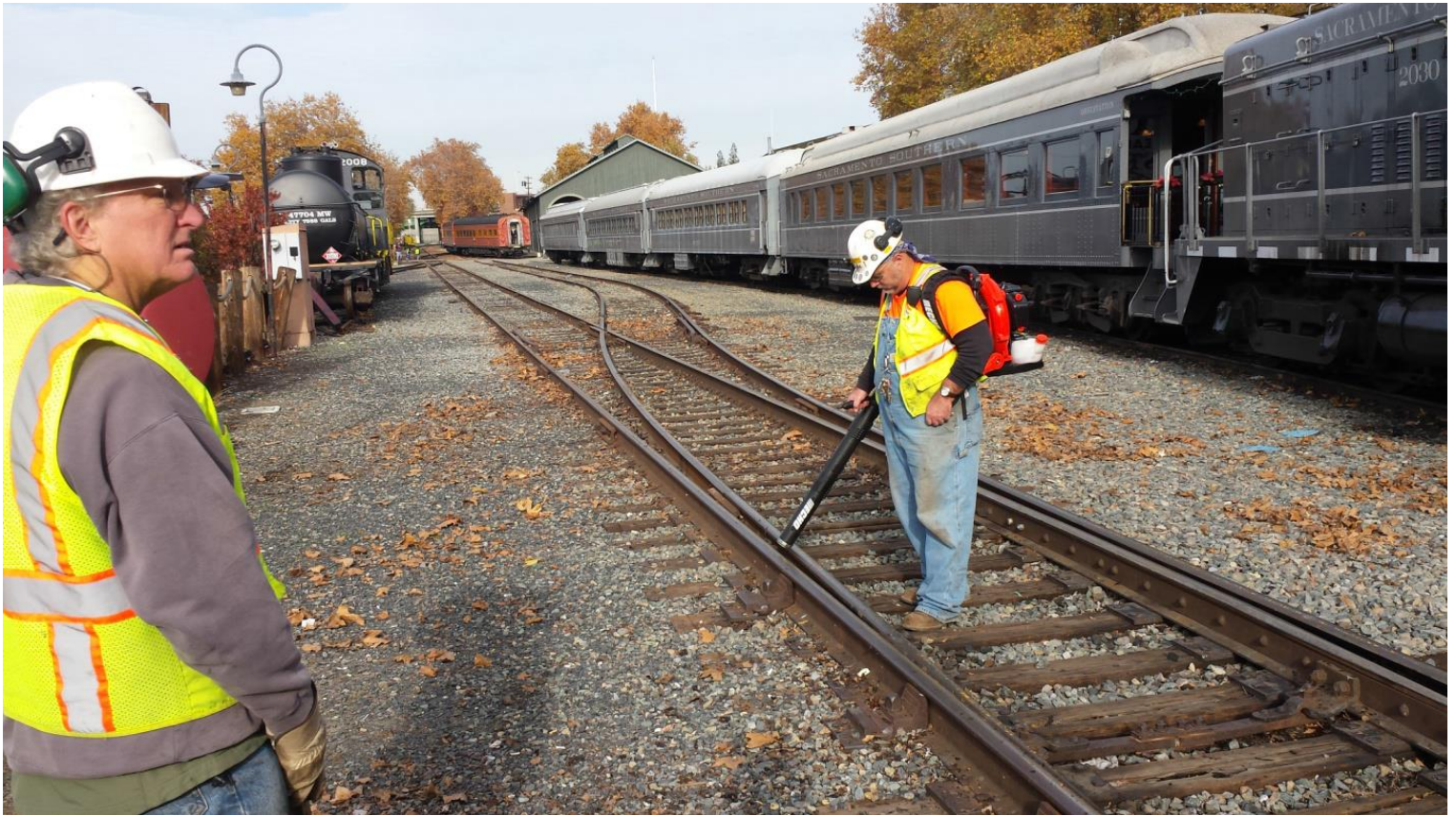
Steve N. looks on while Mike F. uses the huff-'n'-puff machine to eradicate pesky organic debris from Switch 9
